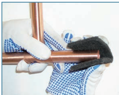
Figure 4: Cleaning of surfaces
