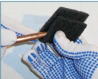
Figure 3: Cleaning the surface
