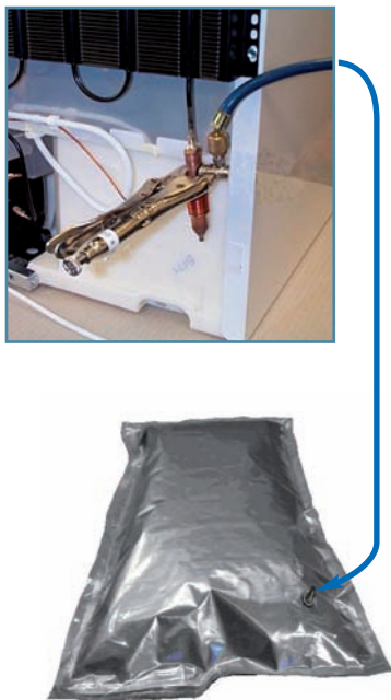
Figure 27: Connecting recovery bag with piercing plier
