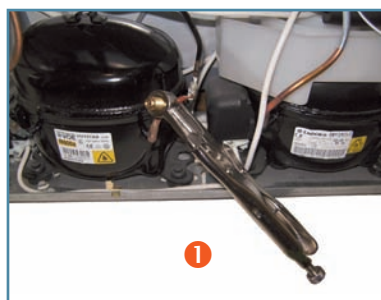
Figure 7: Placement of piercing plier at process pipe
