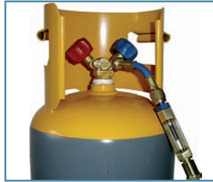
Figure 16: Refrigerant test at cylinder
