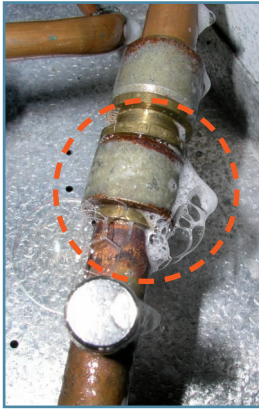
Figure 23a: Example of a leaky connection (see bubbles)
